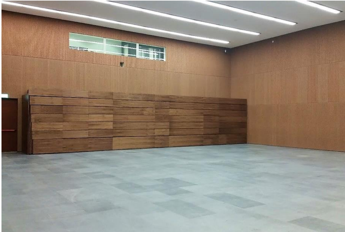
Telescopic folding grandstand [130 seats]
